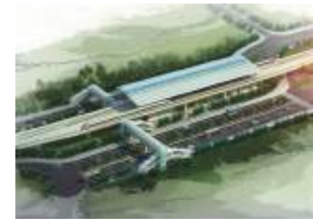
Guangzhou Metro 6 line, Guangdong, China
