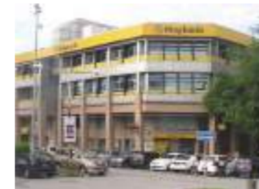
Maybank Damansara Utama, Malaysia
