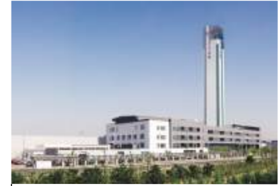
2009, New facility. Landing area:57000m 2 , Construction area:54000m 2 , Test tower height:140m.
