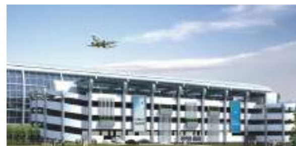
Goa Airport, India
