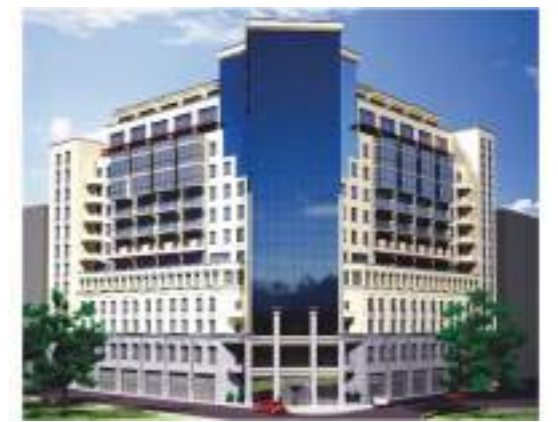
Apart hotel and residential complex, Armenia
