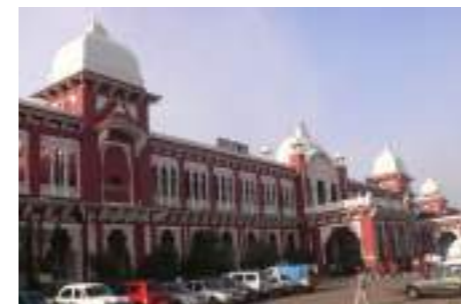
Chennai train station, India
